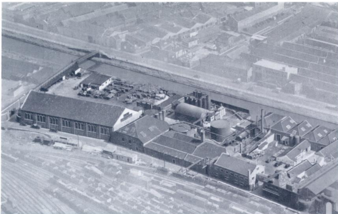
HEAD OFFICE AND STORES, ST. PHILIPS, BRISTOL
