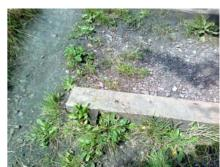
5. Install one timber step approx midway, approx 150cm length. Excavate, regrade and fill to 4m stretch of path, include terram membrane
